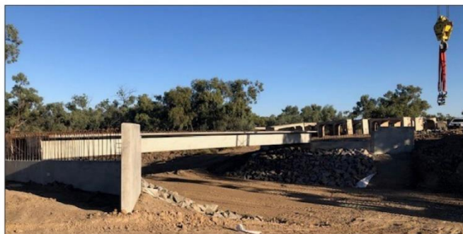
Work has been occurring on the bridge at Yampoola crossing.
