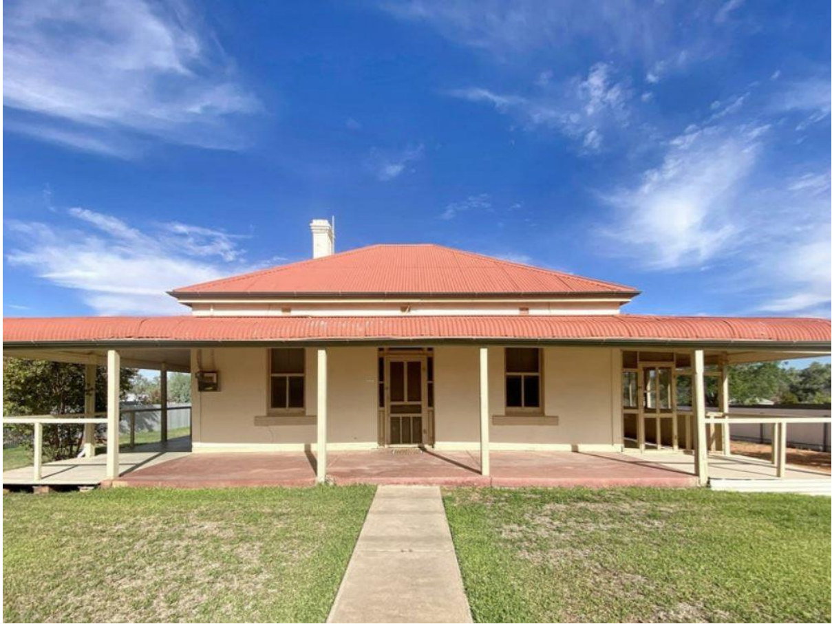
Figure 5: Photo of Lot 32 DP 1064321 from Yartla Street looking South East
