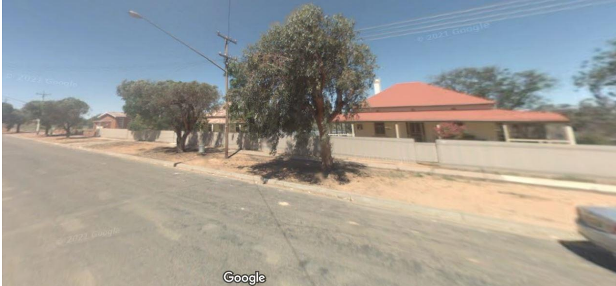
Figure 3: 43 Yartla Street North Eastern View
