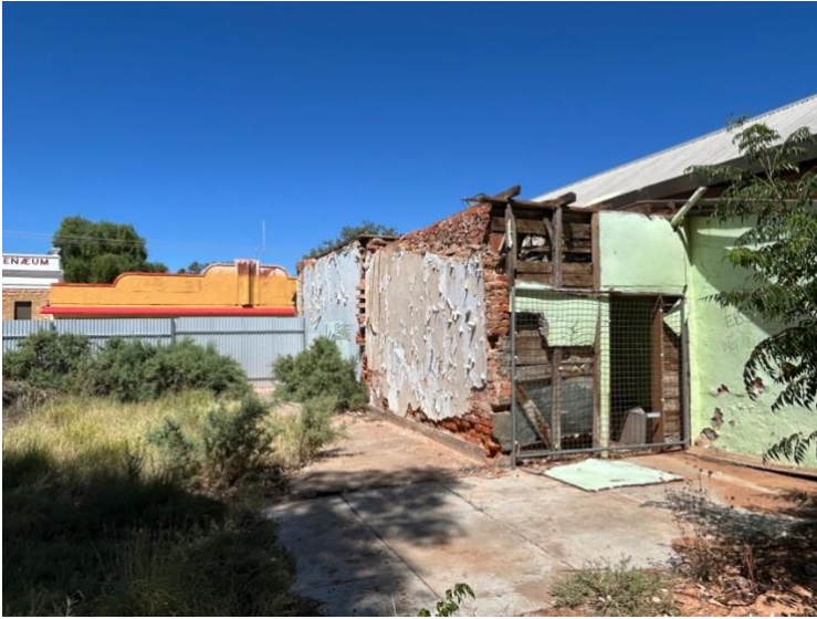
Rear of building section to be demolished.
