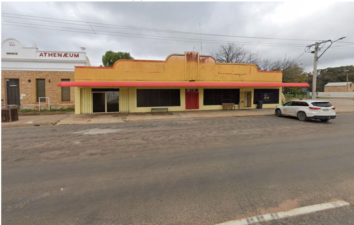
Figure 8 Premises opposite the site - Reid Street Wilcannia Looking South West
