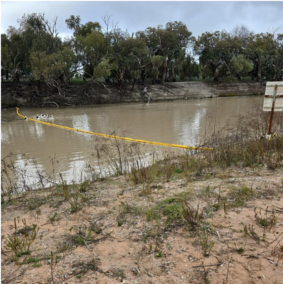
Figure 1: Yellow silt barrier crossing the span of the river.
