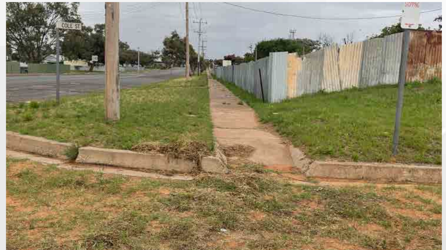
Typical Kerb Ramp Photographs
