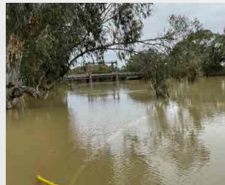
Historic Wilcannia Bridge
