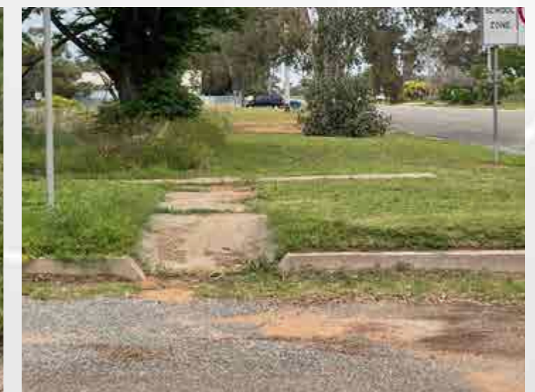
Typical Kerb Ramp Photographs
